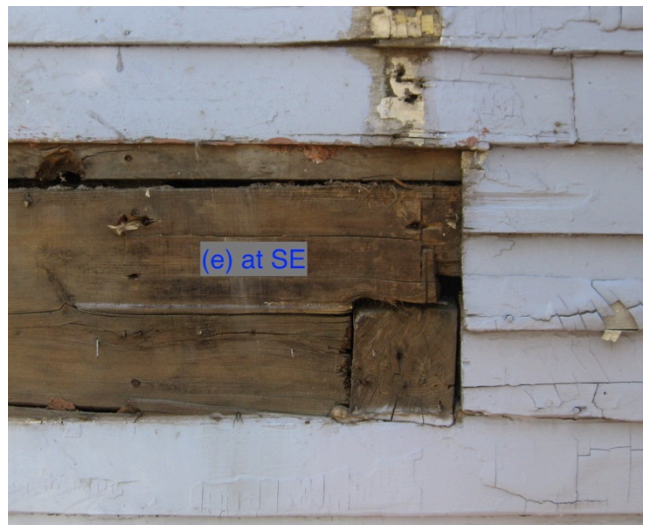
Connection of Second Floor Deck to Main House (DECK 2)
