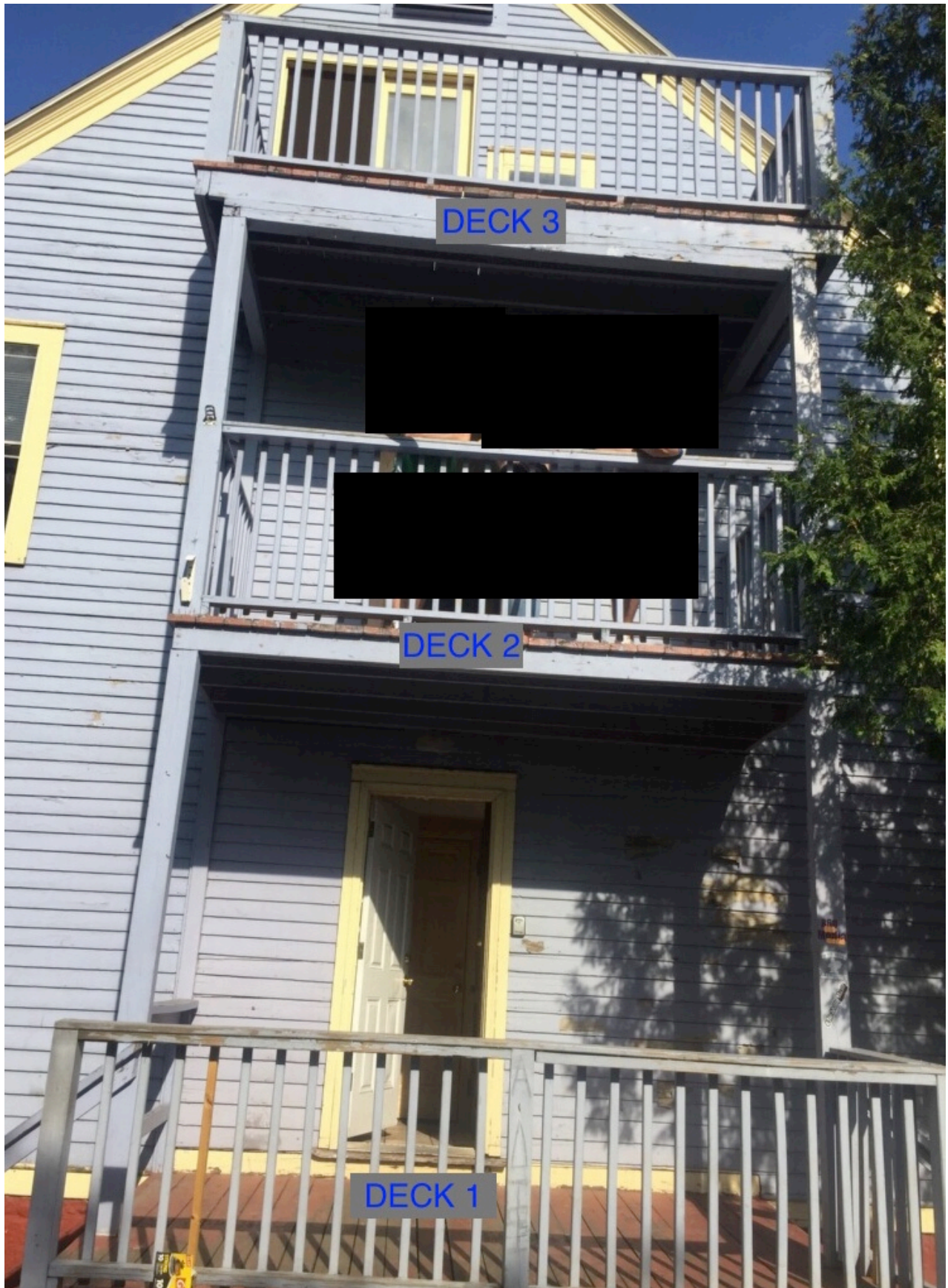
Decks Intact Prior to Failure
