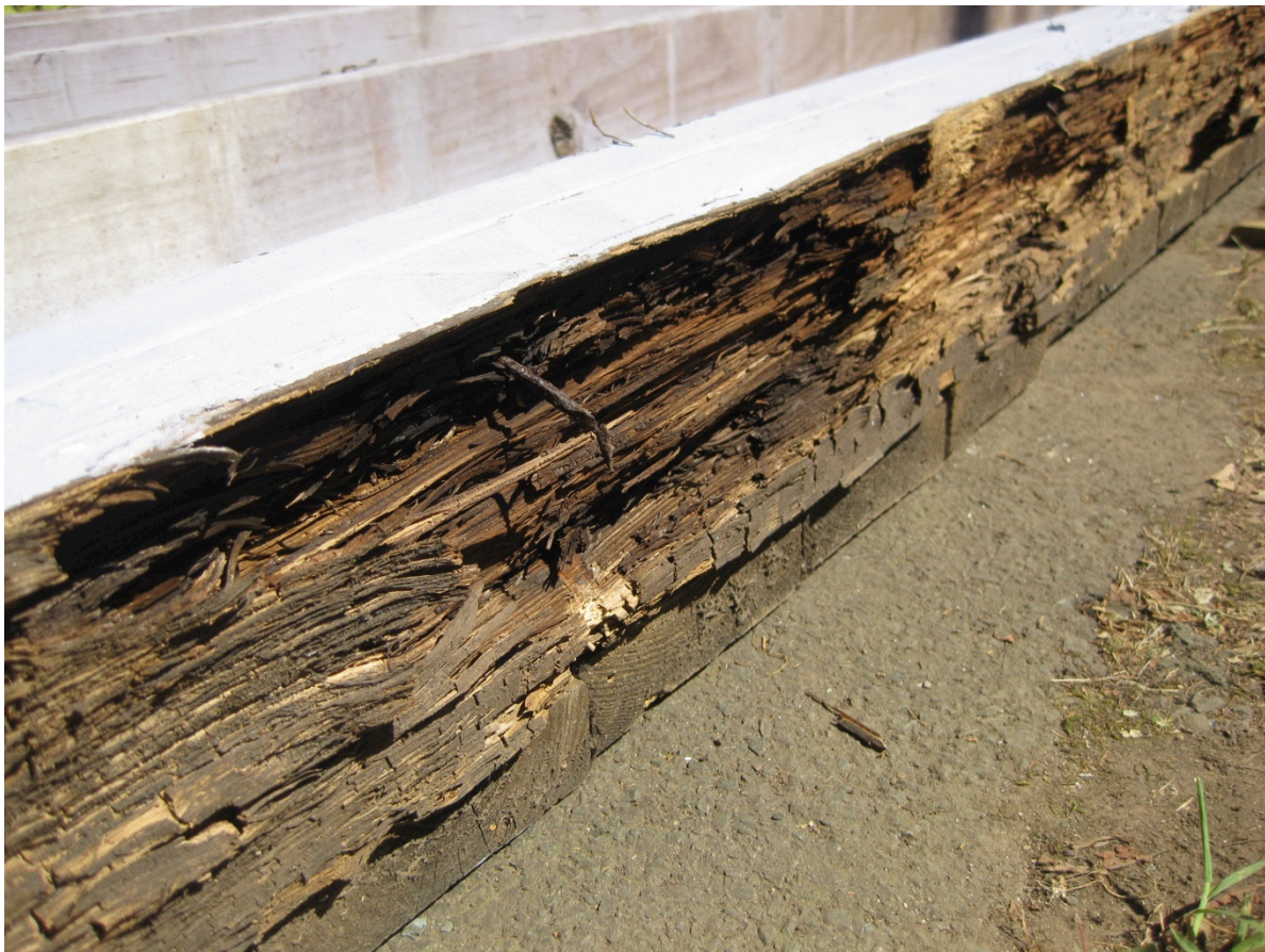
#2. Deteriorated Deck 2 original 1925 ledger and nails
