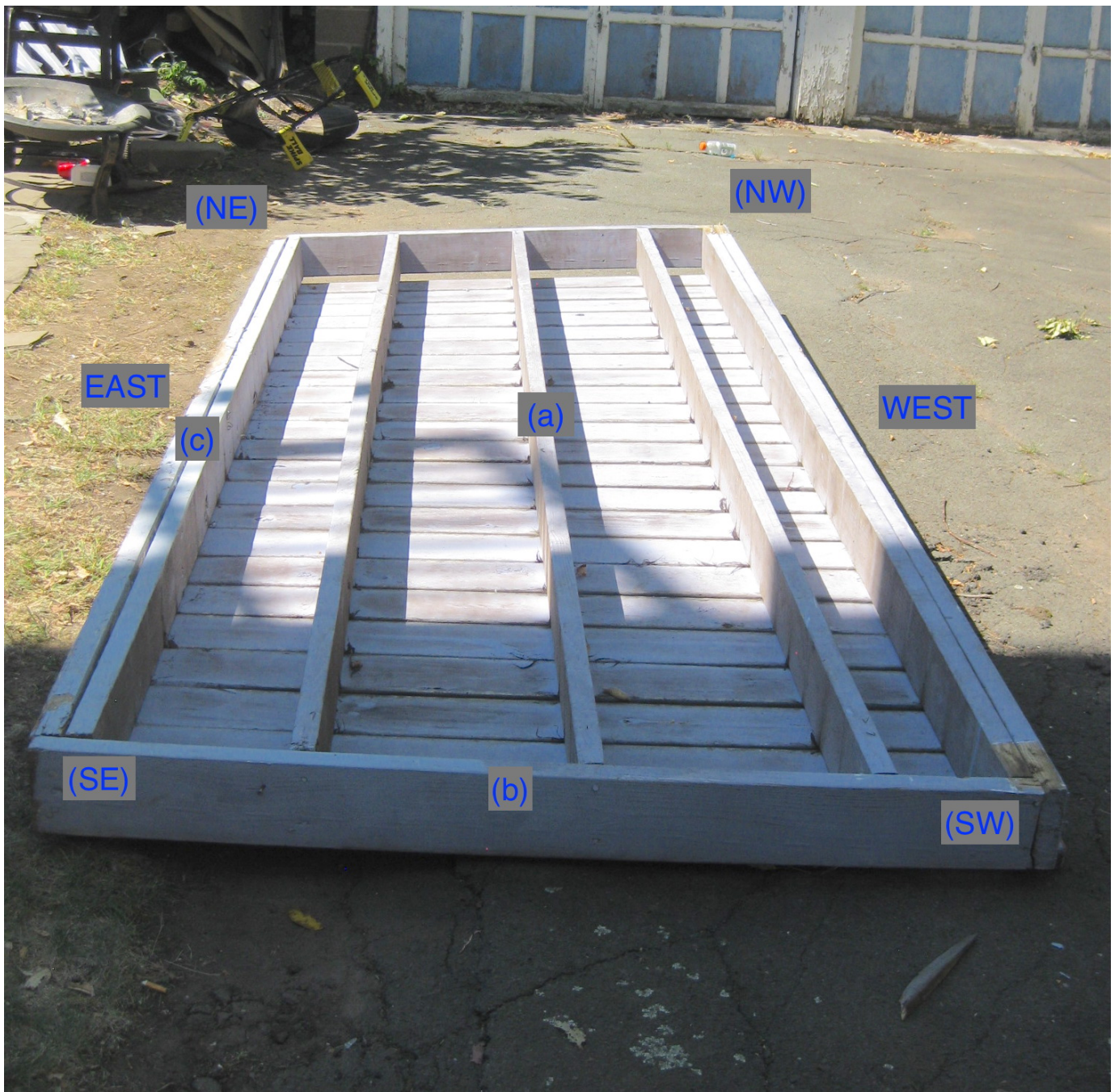
Underside of Second Floor Deck Framing (DECK 2)
