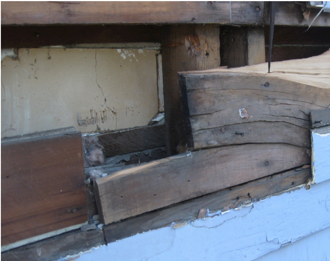
#5. Deck 3, Wall Bearing Support at East End of South Beam
