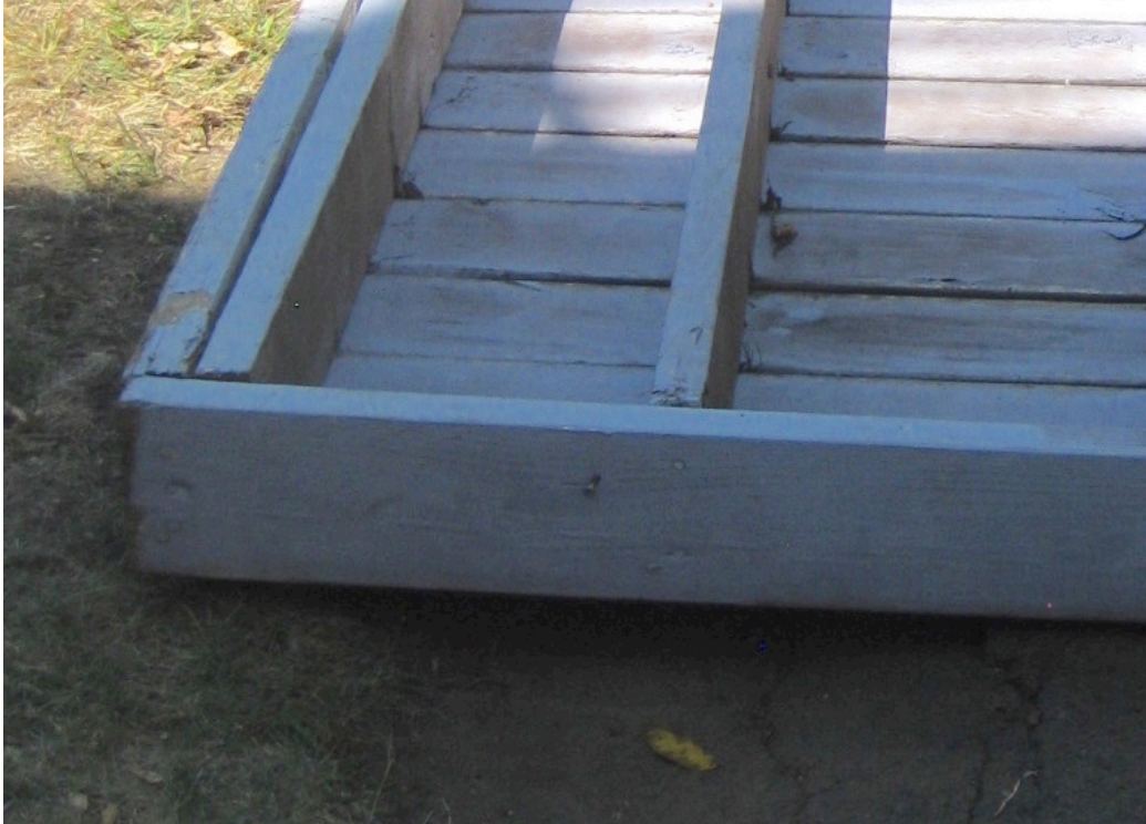
#3. Deck 2 South-East Beam End Connected to Ledger with only 2 nails; SE beam end not extended to bear onto main house wall
