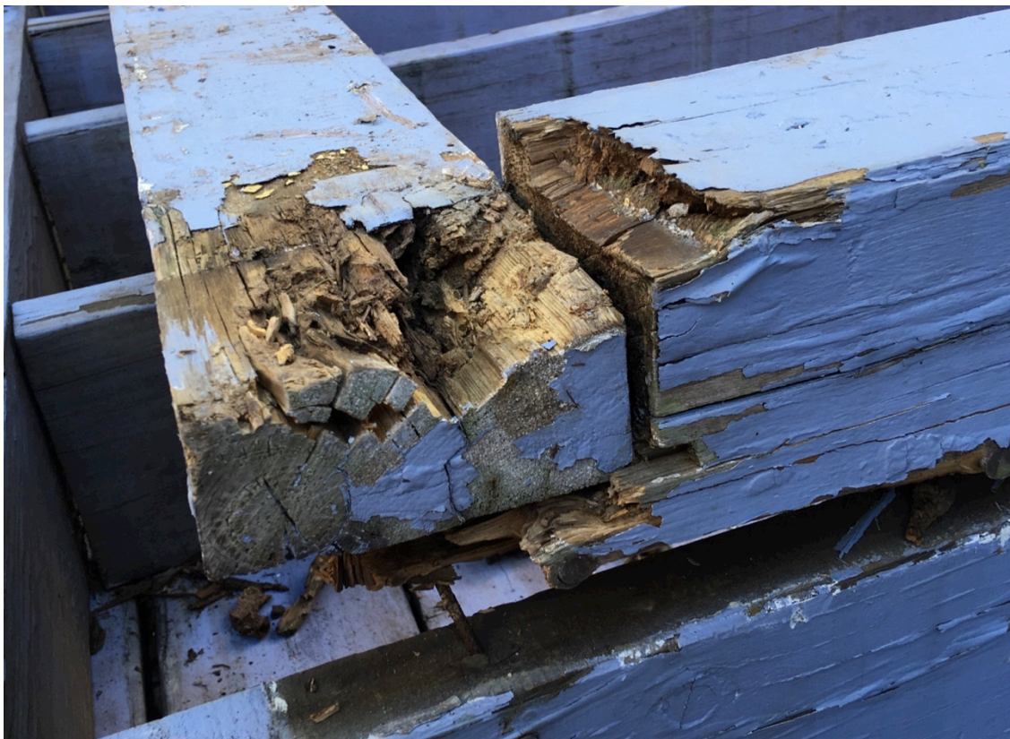
#4. Deck 3 Deterioration at West End of South Beam
