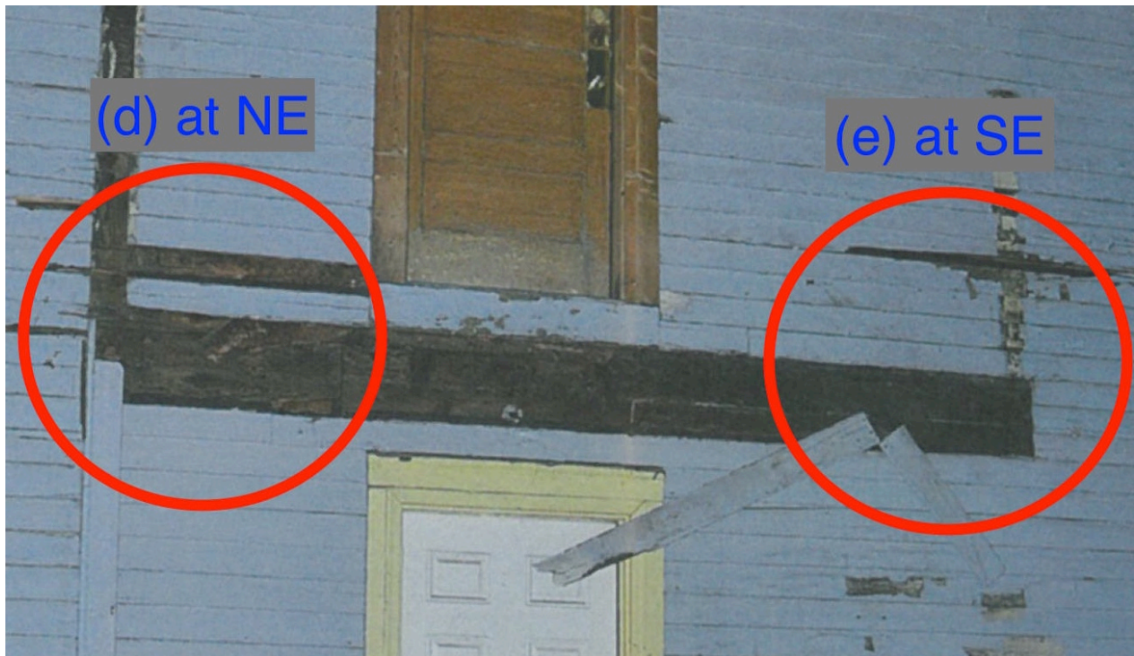
Connection of Second Floor Deck to Main House (DECK 2)
