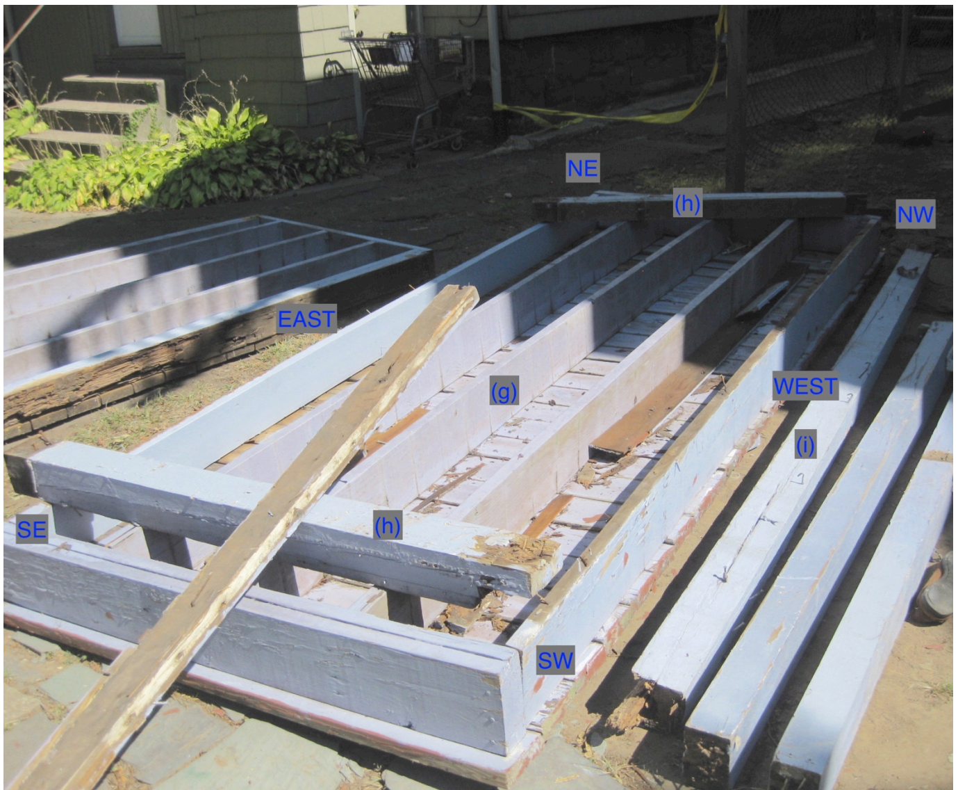
Underside of Third Floor Deck Framing (DECK 3)
